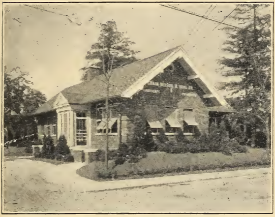
General Offices at Nursery Entrance
